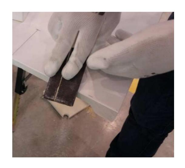
after cutting and before installation, carefully sand the cut edges with sandpaper to slightly round the edges
